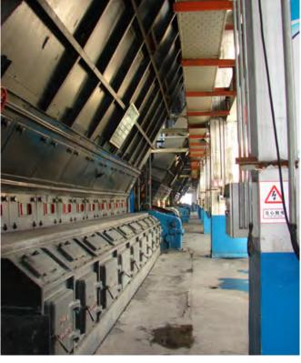
8 units of 70 MW high temperature hot water boilers and auxiliary engines installed in the project.
