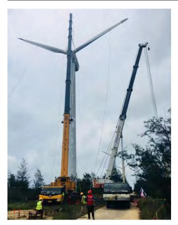
Installation process of German NORDEX N43/MK3 fan.
